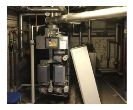
Watsons Building Services Ltd completed a phased project involving the removal and replacement of old boiler and hot water plant systems and controls. The project also encompassed electrical works and integration with a Building Management System.
