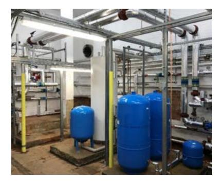
We successfully tendered the installation of a new boiler plant and advanced controls, specifically tailored to serve the 'old building' nestled within the college grounds. This project was initiated due to the realisation that the existing remote boiler plant, catering to the 'new building,' fell short of delivering sufficient heat to meet the heating demand.
