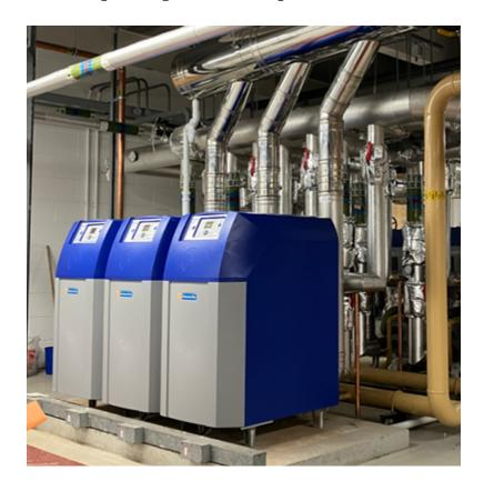
The project involved the complete overhaul and replacement of a Gas-Fired Boiler System with new state-of-the-art Condensing Boilers. We designed, installed, tested and commissioned six new gas-fired boilers, including stripping out and removing the old boilers and pipework, installing new gas pipework, flow and return pipework, and installed a dedicated flue system which vented to atmosphere.
