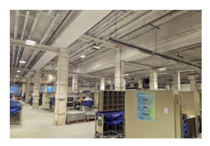
The project involved the upgrade and replacement of a series of gas-fired warm air heaters at a Factory and Distribution Centre. This project also included the design, supply, installation and commissioning of additional Radiant Tube heating systems to areas of the warehouse.
